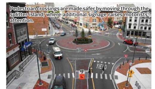
Pedestrian crossings are made safer by moving through the splitter island, where additional signage raises motorists' attention.
