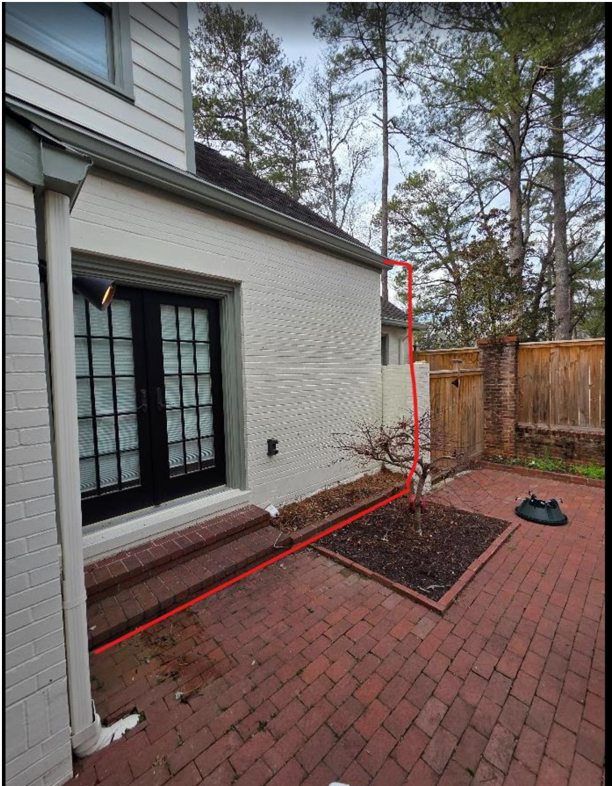
Figure 5 – Small extension to provide more square footage and provide room for the door to the new bathroom
