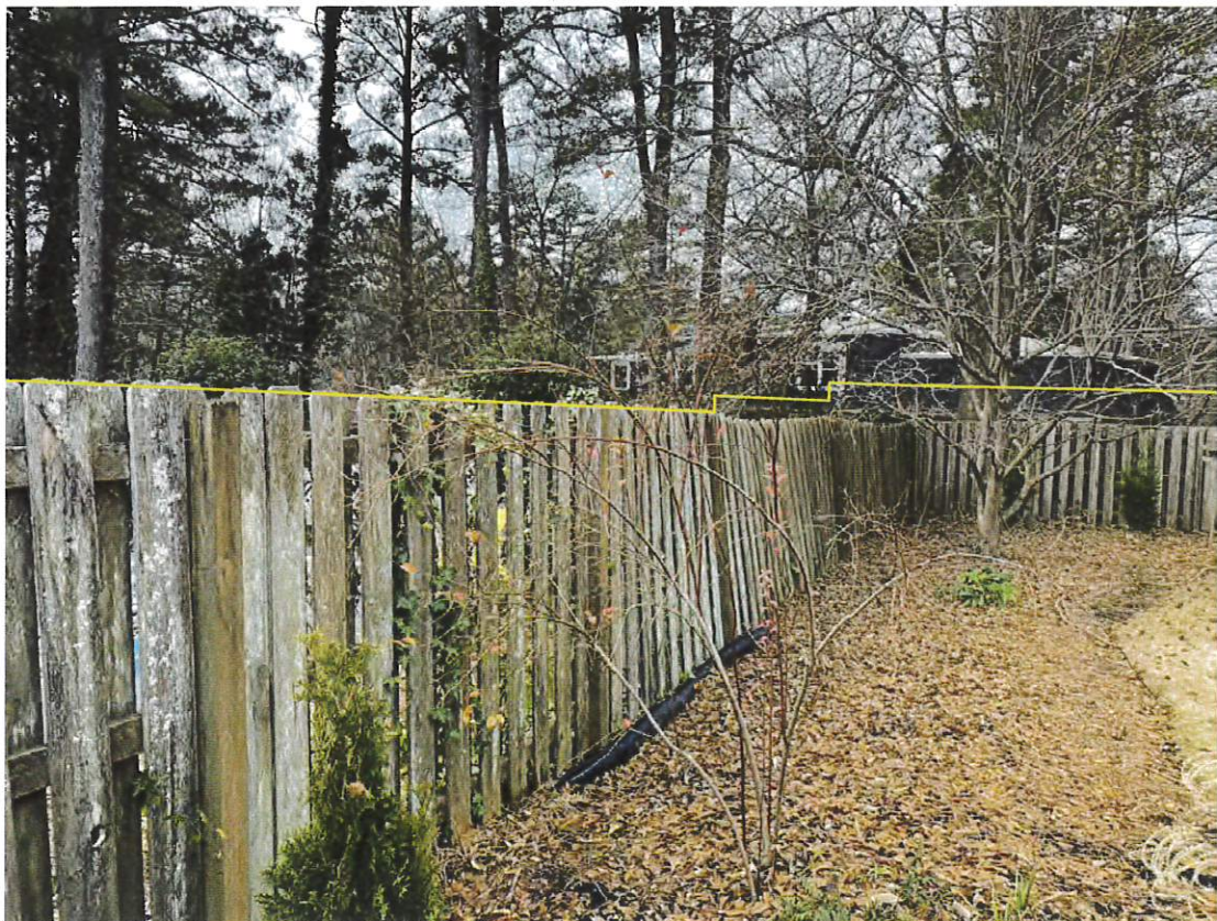
Above: View looking approximately West toward the houses on Lakeview Plaza. Line shows change from a 6' height on the right, gradually increasing to 8' at the far left. Below: View looking along the NW edge looking approximately NW toward the houses on Lakeview Plaza. Line shows stepped height starting at 6' at the left, increasing to 8' approaching the corner at the bottom of the grade.
